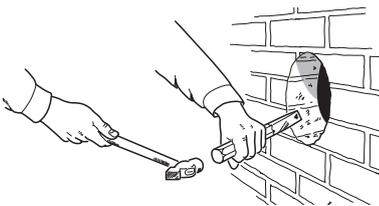
Mark out centre for making a hole in the wall to the flue. Check that the connection height in the chimney breast corresponds to the height of the connection pipe from the stove.
